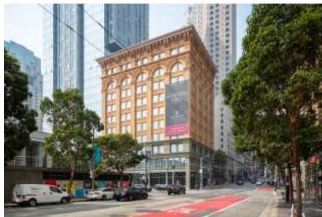
The Aronson building
