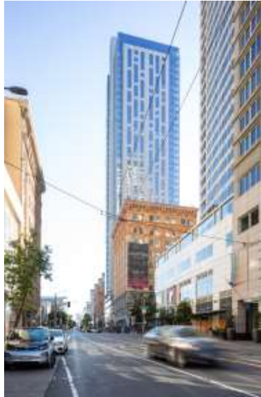
Four Seasons Private Residences at 706 Mission as viewed from beside the Museum of the African Diaspora.
